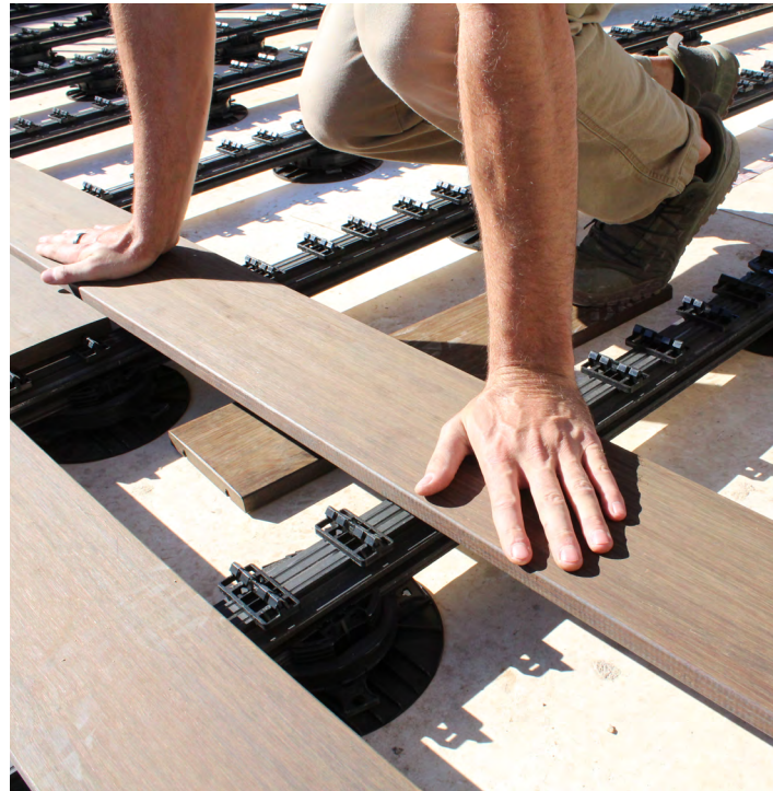
↑ Grad® Decking Installation
