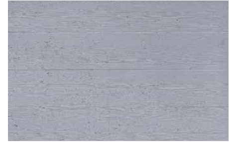
COFFRAGE FORMWORK Studio LCDA
