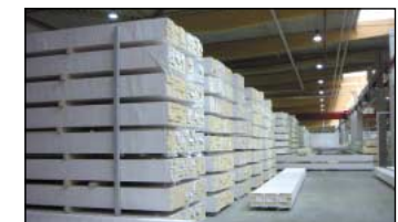
Largest glulam warehouse in Europe
